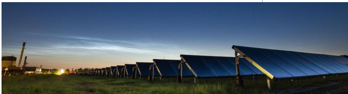
Løgumkloster district heating facility with a solar panel park compromising 15 300 sqm.
